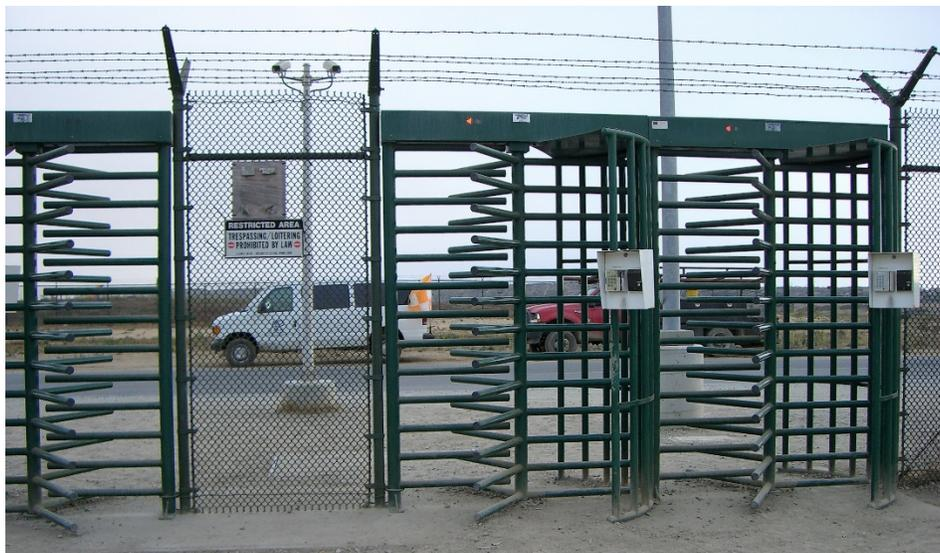
The two turnstiles on the right-hand side are landside-to-airside gates. They only turn one way, have access control readers on the gates, and are monitored by CCTV cameras. The left-hand side gate is an exit gate. The gates are topped by barbed wire and about 8-foot high fencing.
